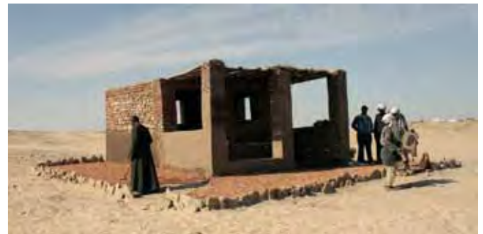
Figure 15. New shed for the guards, built in 2011
